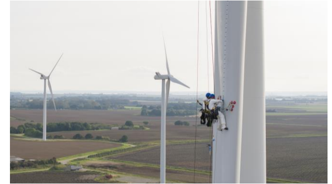
Vortex generator install
