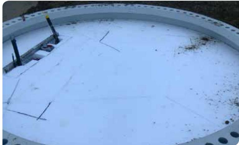
Figure 15. Insulated wind power foundation.
