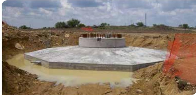
Figure 2. Example of gravity foundation under construction.
