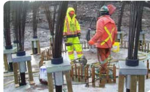
Figure 3. Example of rock anchored foundation under construction.
