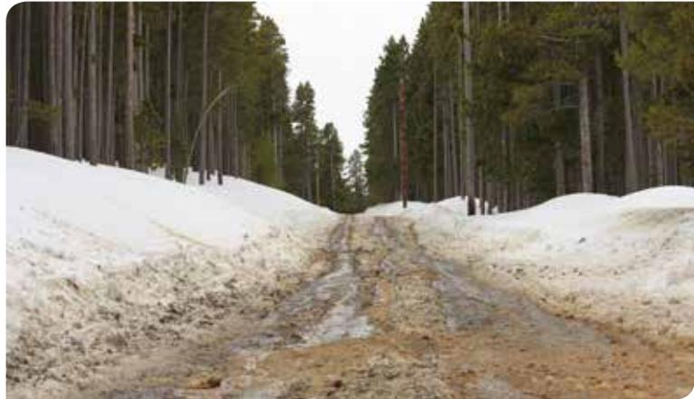
Figure 10. Thaw weakening of a gravel road.
