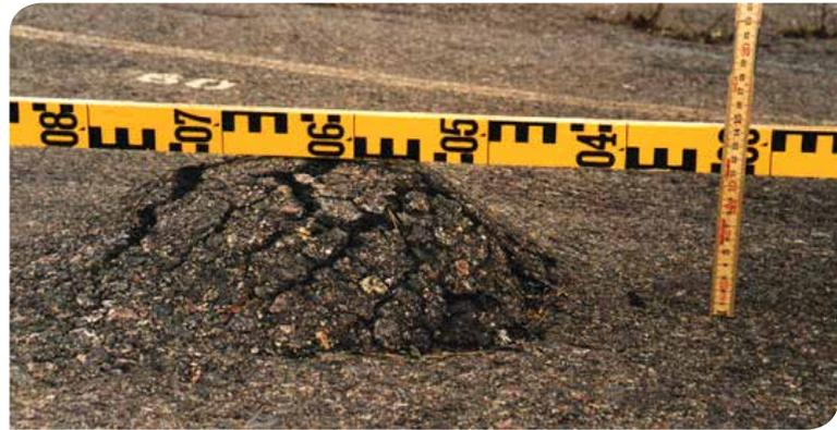
Figure 9. Example of stone lift under pavement caused by frost heave.
