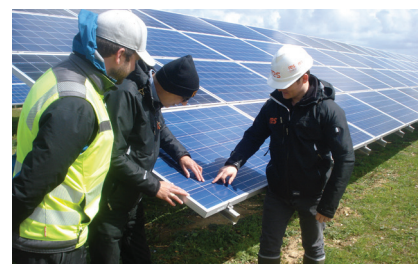
Inspecting micro crack evidence
