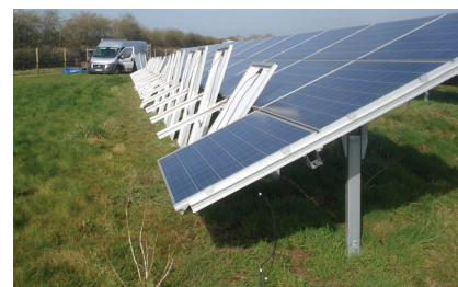
On-site panel performance testing
