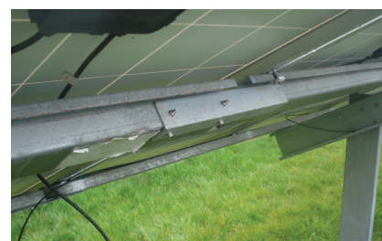
Thermal expansion joints inserted
